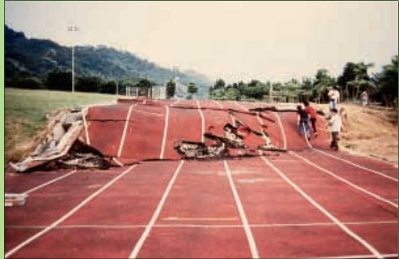
◆ FIGURE 4 One hundred yard . . . dash? The September 21, 1999 earthquake ( M_w = 7.8 ) in Taiwan was caused by movement on the Chelungpu fault. This running track at Kuang Fu High School was built across the fault that here had a vertical offset of 2.5 meters (8.1 ft). It is obvious that no 100-meter-dash records will be broken here.
