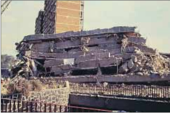
◆ FIGURE 4.13 (Total vertical collapse as a result of “story shift”; Mexico City, 1985. Such structural failures are not survivable.
