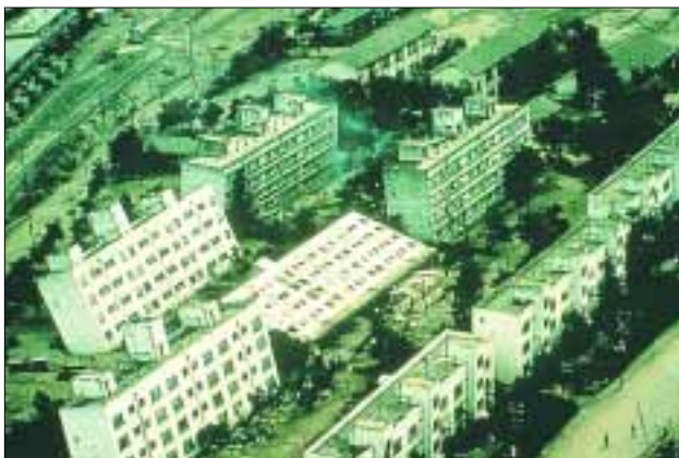
◆ FIGURE 4.16 (a) These apartment buildings tilted as a result of soil liquefaction in Niigata, Japan, in 1964. Many residents of the building in the center exited by walking down the side of the structure. (b) “House of cards” collapse of quick clay structure in Turnagain Heights, Anchorage, Alaska in 1964. Total destruction occurred within the slide area, which is now called Earthquake Park.
