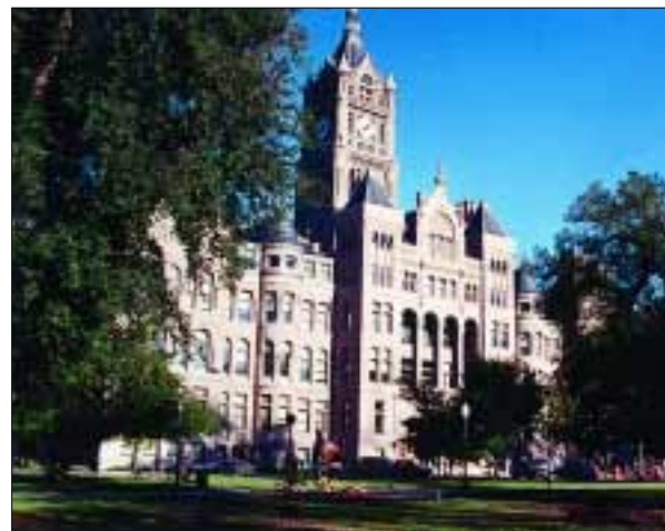
◆ FIGURE 4.39 Salt Lake City and County Building, Utah. Constructed in 1890, largely of brick, it is now seismically retrofitted to meet the modern building code.
