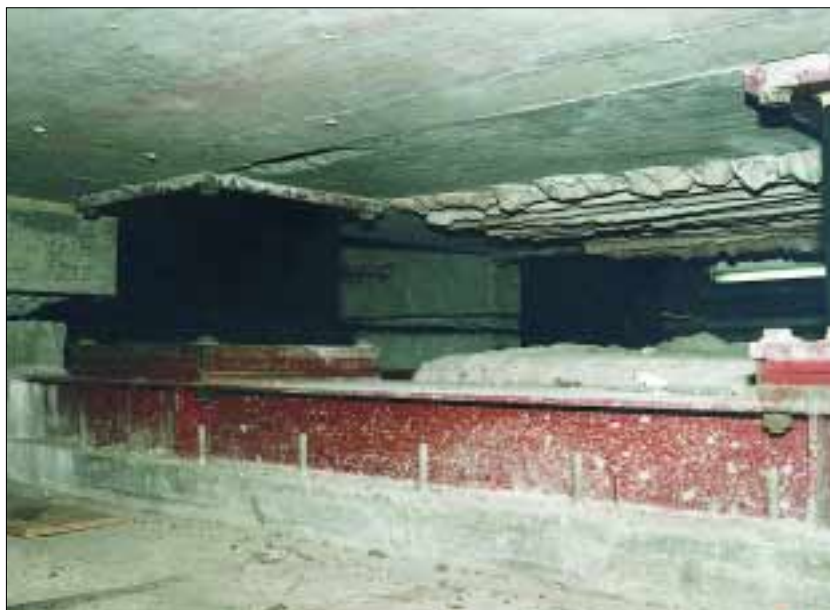
◆ FIGURE 4.40 Basement of the Salt Lake City and County Building. The building has been seismically retrofitted by cutting the massive structure from its foundation pillars (one shown on the far left, another in the center of the photograph), and lifting the building onto 440 large rubber isolators (one left of center, another at the extreme right of the photograph).
