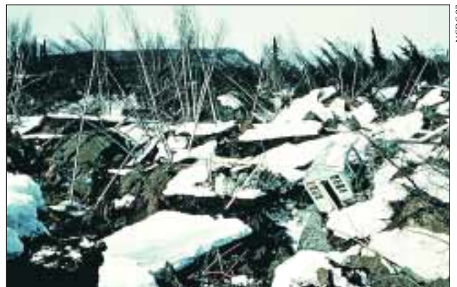
◆ FIGURE 4.16 (a) These apartment buildings tilted as a result of soil liquefaction in Niigata, Japan, in 1964. Many residents of the building in the center exited by walking down the side of the structure. (b) “House of cards” collapse of quick clay structure in Turnagain Heights, Anchorage, Alaska in 1964. Total destruction occurred within the slide area, which is now called Earthquake Park.
