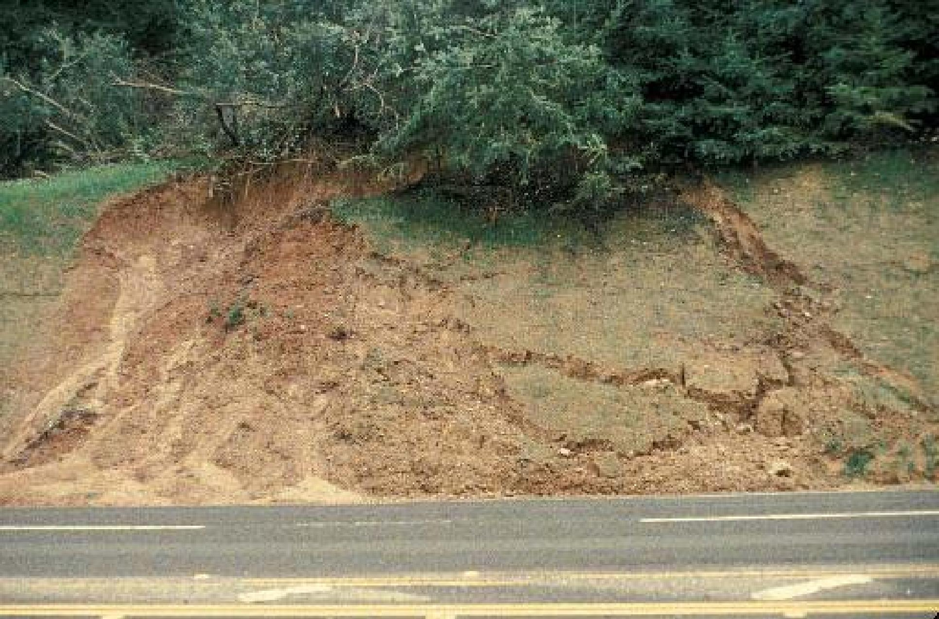
This photograph shows two types of sediment failure next to each other. A landslide and a debris flow have occurred at the same time in this eight meter high California roadcut in rain saturated soil. The difference in water content may account for the two types of failure.
